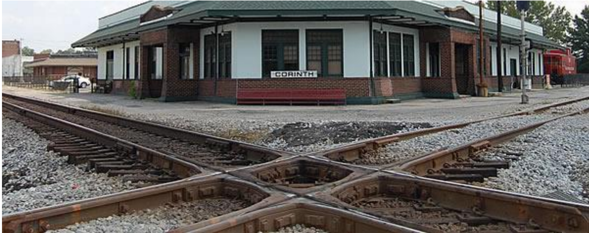
The railway junction at Corinth
